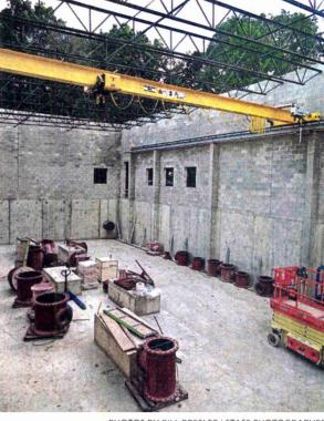
PHOTOS BY BILL BRESLER | STAFF PHOTOGRAPHER The pumping station controls the flow of water. The three-ton overhead crane helps with replacement of motors,
